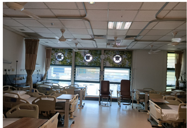
Rapid retro fitting completed in TTSH wards
